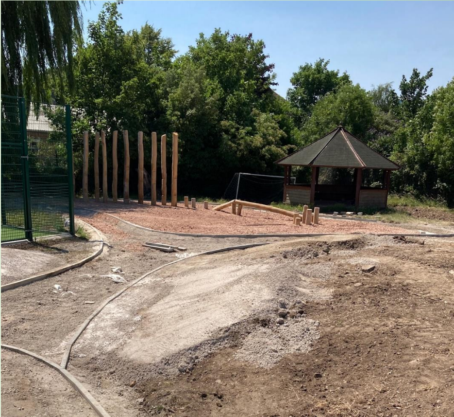
Autonomous area with balance beams and traversing poles in place
