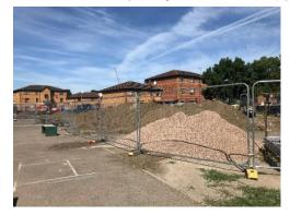
compound and are now preparing the ground for the new climbing frames that replace the trim trail. This involves digging down 600mm to get out the roots of all the old trees that had to be cut down in the past few years. They have also started to dig the running track around the edge and will soon
